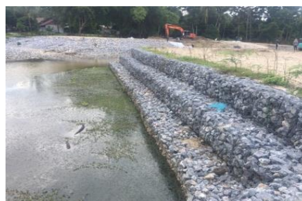
Constructed bank protection wall
