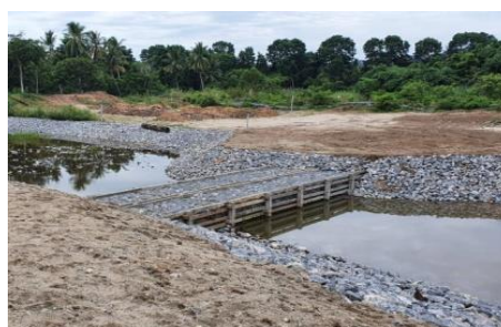
Constructed sediment detention weir
